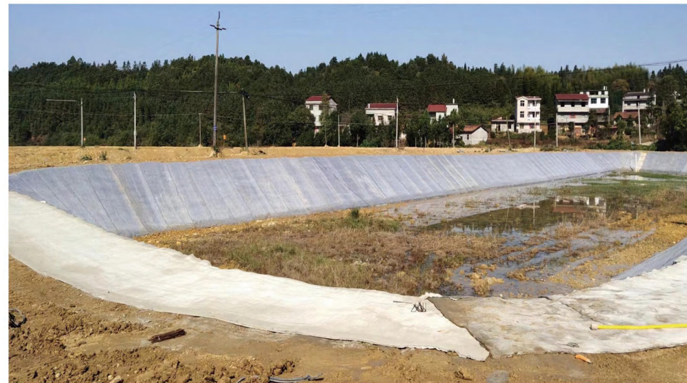
河塘沟渠 River pond ditch
